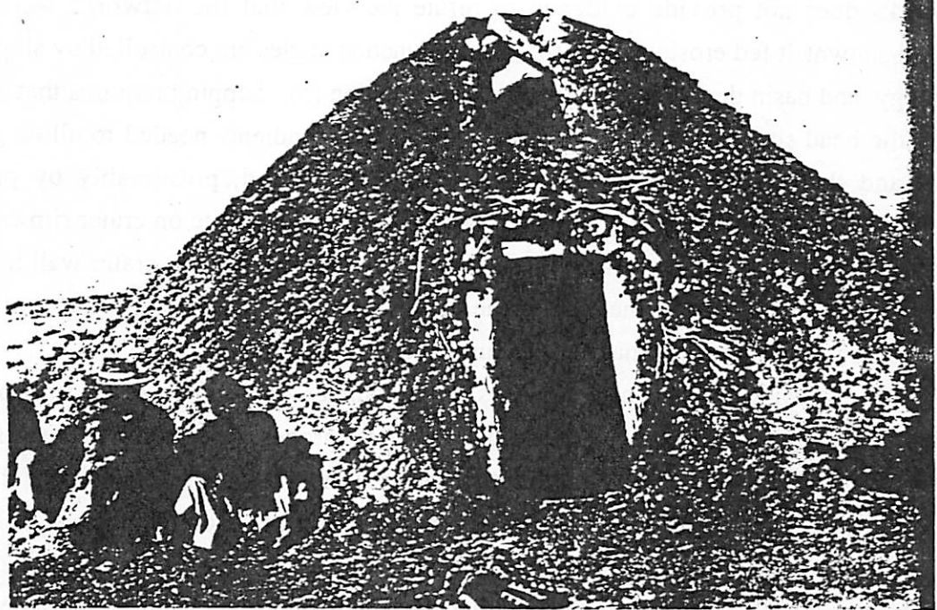
A forked-stick hogan, the type of dwelling used by the earliest Navajos. (Photograph by Milton Snow, Courtesy U. S. Indian Service)
