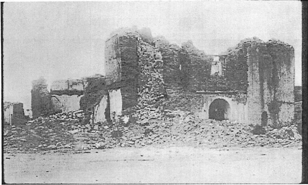
Fig. 4 - A building in Bavispe, Sonora, Mexico, destroyed during the 03 May 1887 earthquake.
