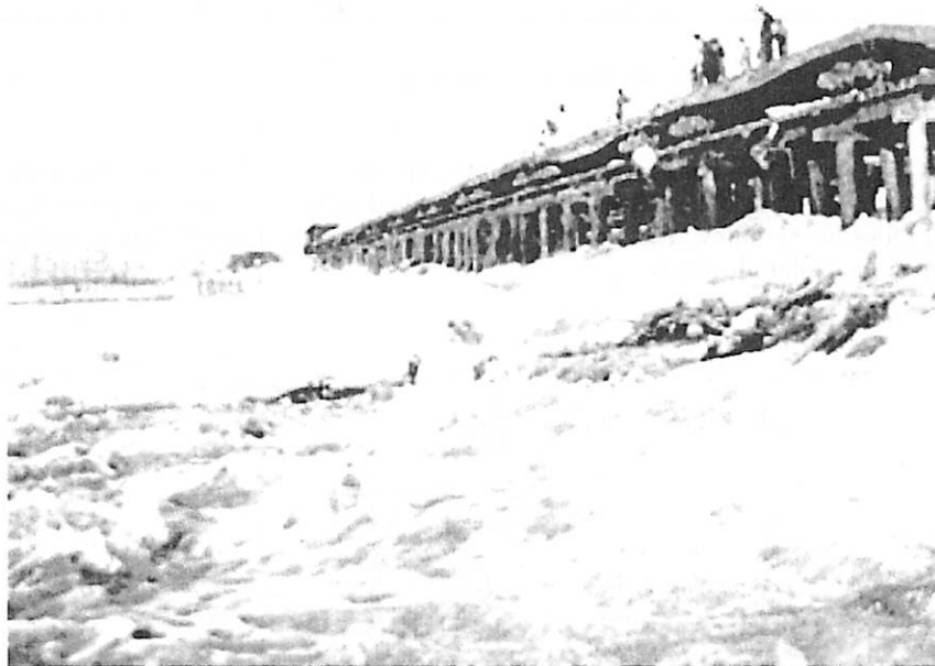
FIG. 2 Flooding of the canal overwhelms the poorly built controls on the flow. (2)
