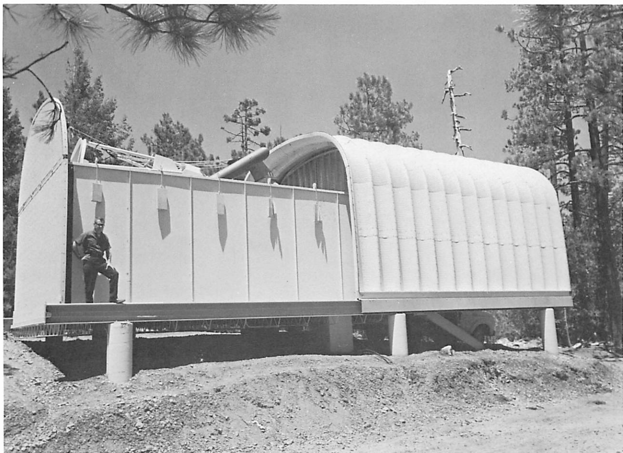
Fig. 8 The roll-off-roof building which houses the 60-inch photometric telescope. The telescope is shown in its rest position. The south wall of the building (at left) is hinged and folds down for observations of southern stars. The hanging weights counterbalance the wind screens.
